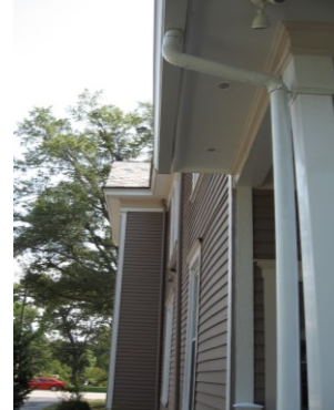
downspouts replaced
